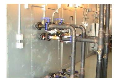
While the use of grooved piping is accepted by the industry for these applications, it's impossible to inspect the joints to ensure ongoing integrity once piping is installed and fully insulated without removing and later re-installing the piping insulation. Over the past several years, the NIH Campus has experienced several high-profile failures of grooved piping joints on chilled water and heating water applications. These failures resulted in
