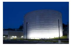
> The Thermal Energy Storage System (TESS) increases energy efficiency by producing and storing chilled water during off-peak hours, which can then
