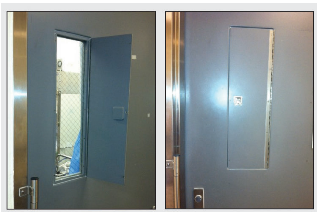
Figure 4.2.3.8 ARF Door Vision Panels and Hardware
