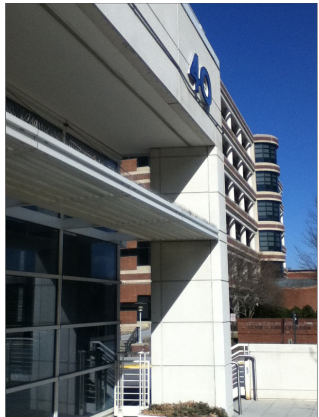
Figure 4.1.6 Sunshading at Building Entrance
