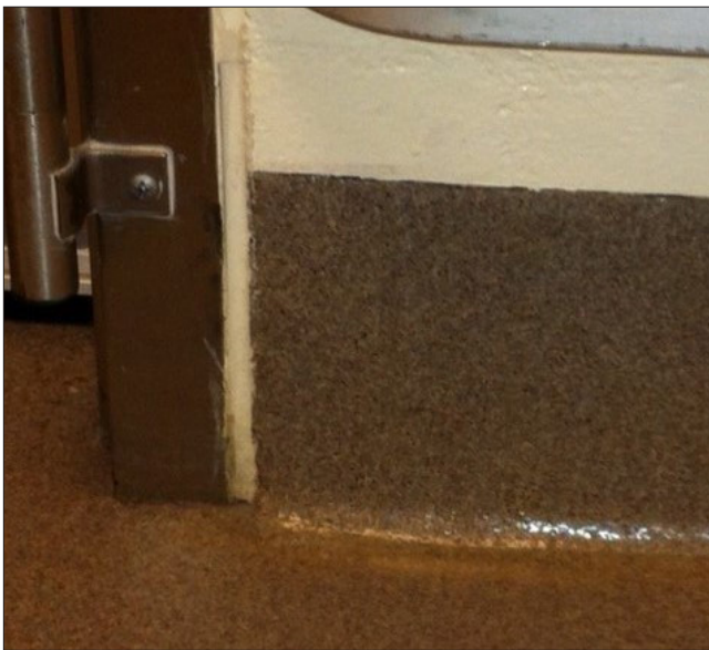
Figure 4.4.4.2.2 Integral Cove Base Detail
